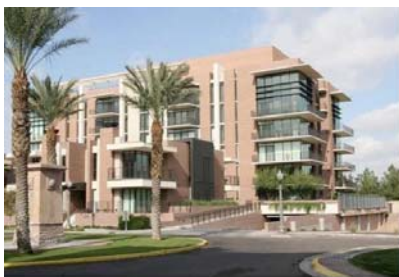
Portland Place on W Portland, Phx
